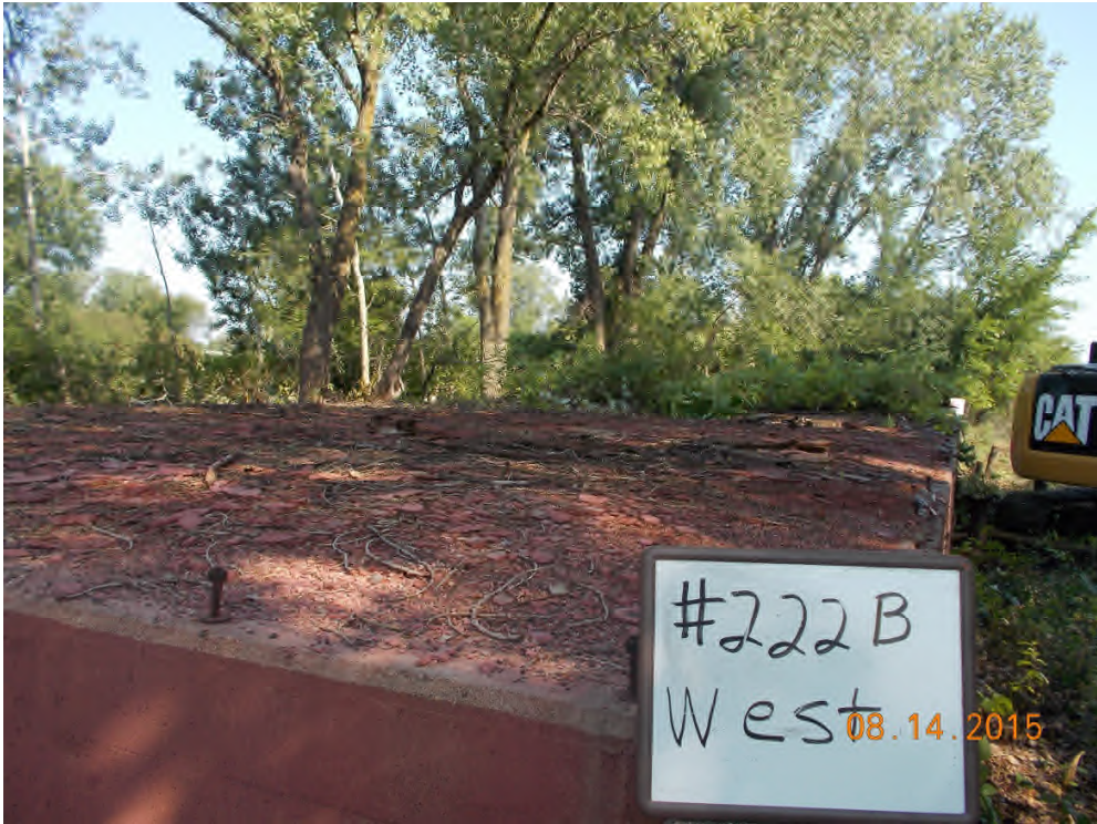
Foundation #222B west before cleaning
