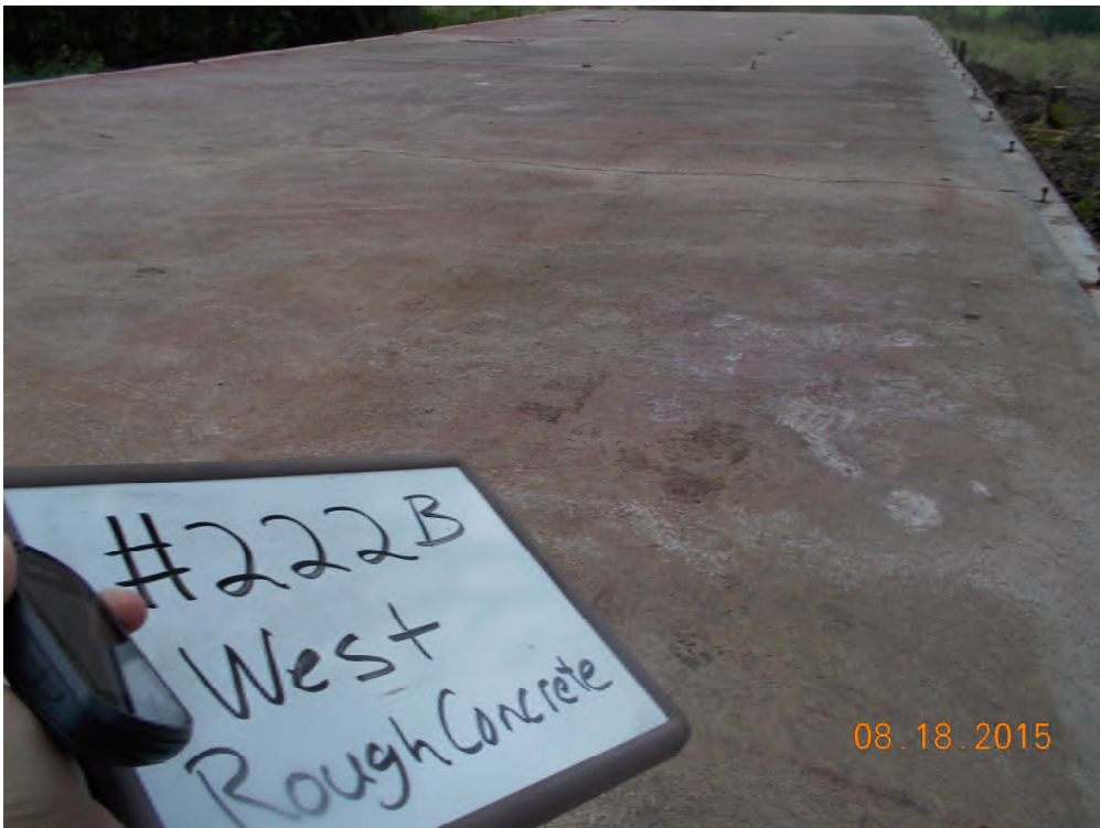
Foundation #222B west after cleaning
