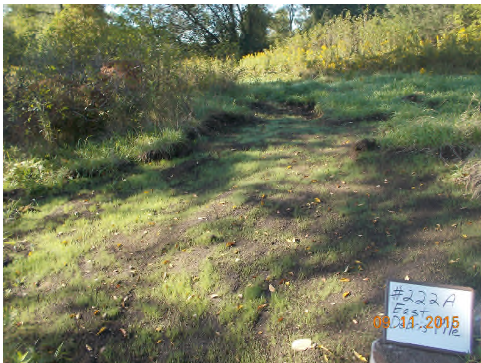
#222A East debris pile south of foundation after excavation and seeding
