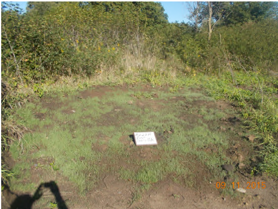
#222A East debris pile northwest of foundation after excavation and seeding
