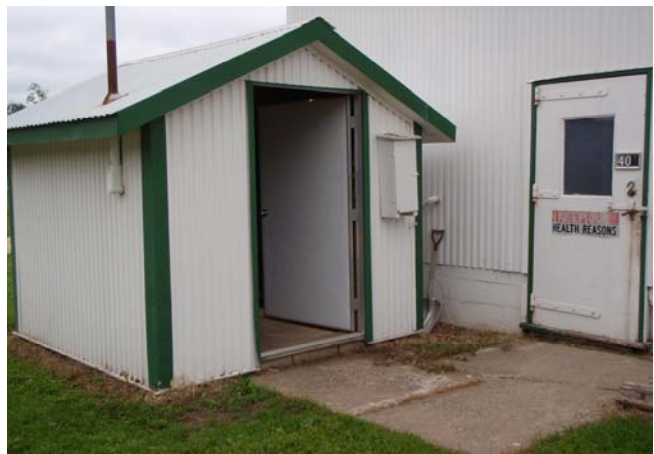
Pump House for Well 207616
