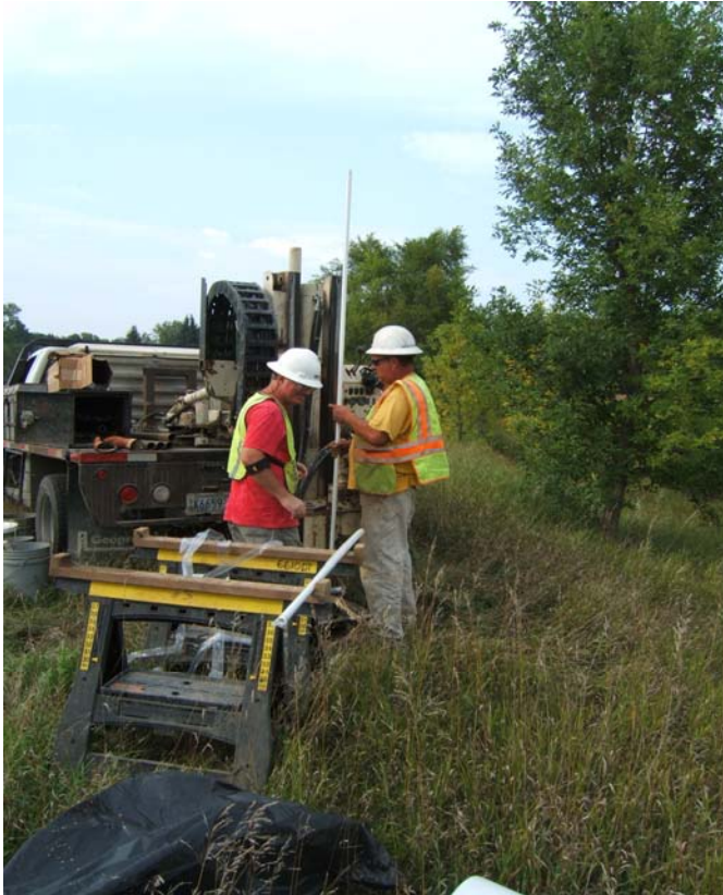
Photo 13 Temporary well installation at SOC4-GP1
