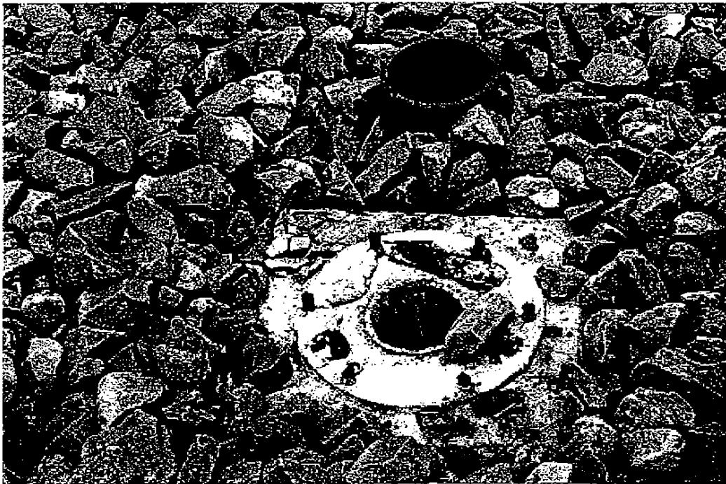
MSP-70, Trickling filter pedestal - mercury bearing absent.
