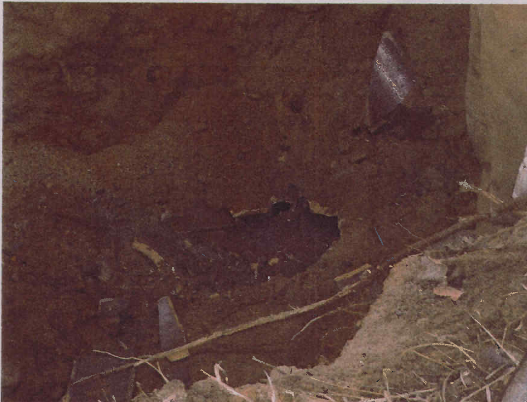
Nitric Acid Plant Area. View of test pit NA-TP-3, which was completed around a brick structure which accessed a buried clay drainage line associated with former above ground acid storage tanks.
