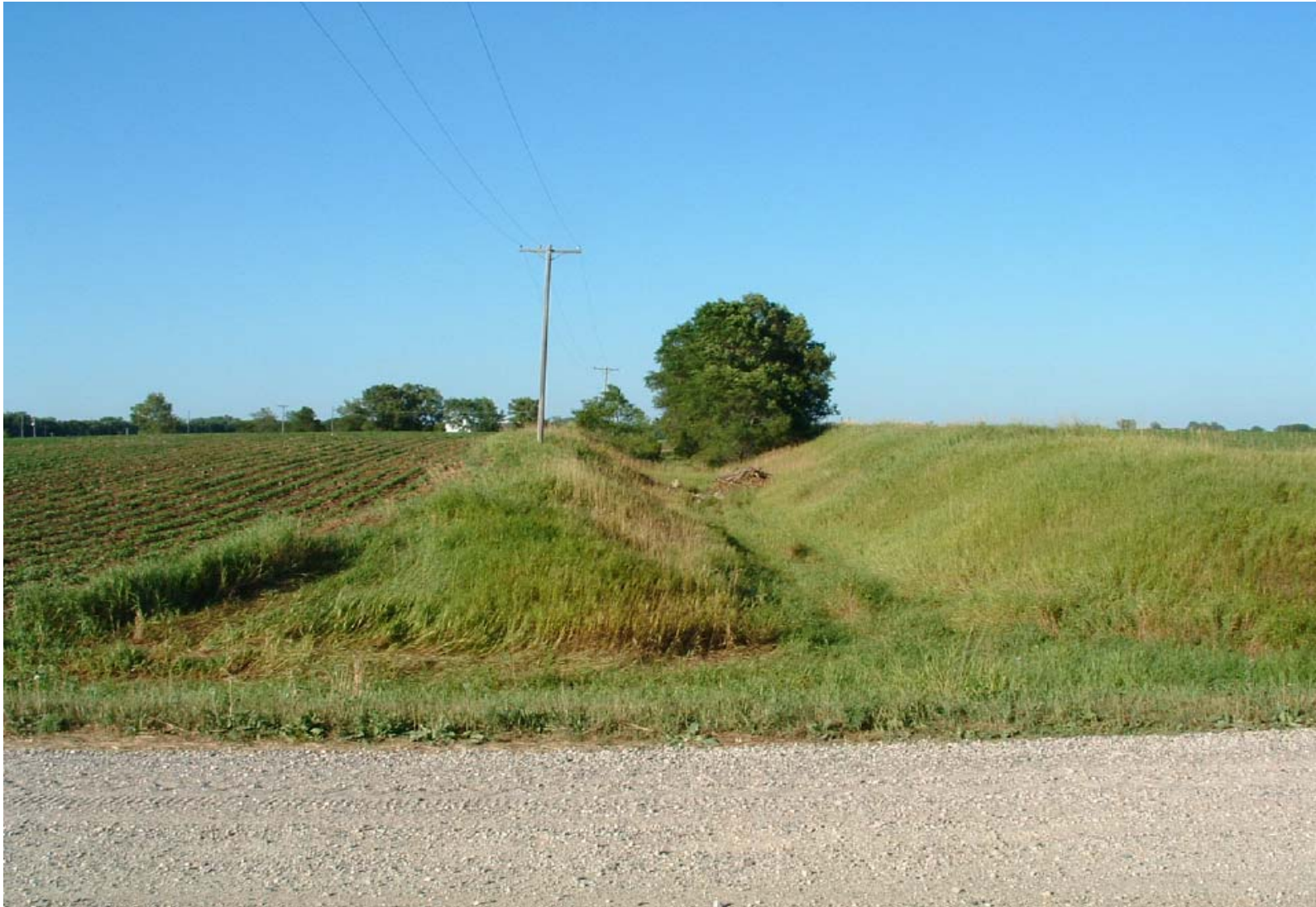
Photograph 11: Drainage Ditch South of DNT Bunkers Looking to the Northwest
