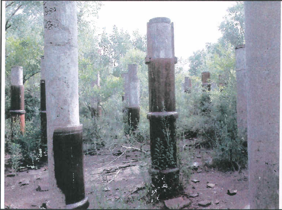
Photo 1: 108-F Boiling Tub House - Columns with ceramic tile coating
