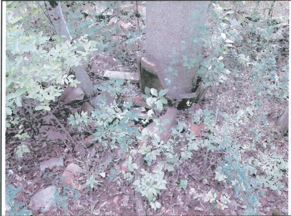
Photo 15: 108-B Boiling Tub House column
