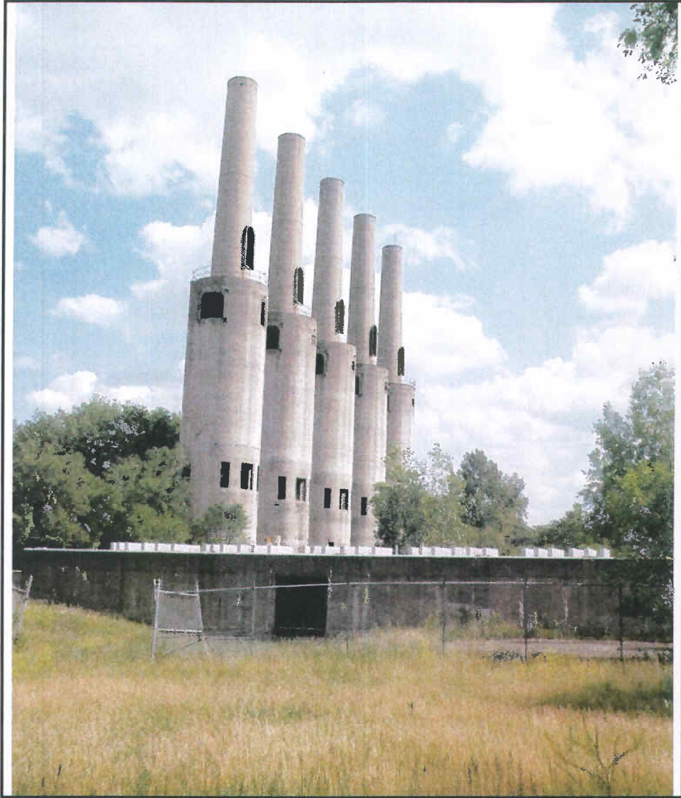
Photo 31: Five remnant stack structures associated with Power Plant A
