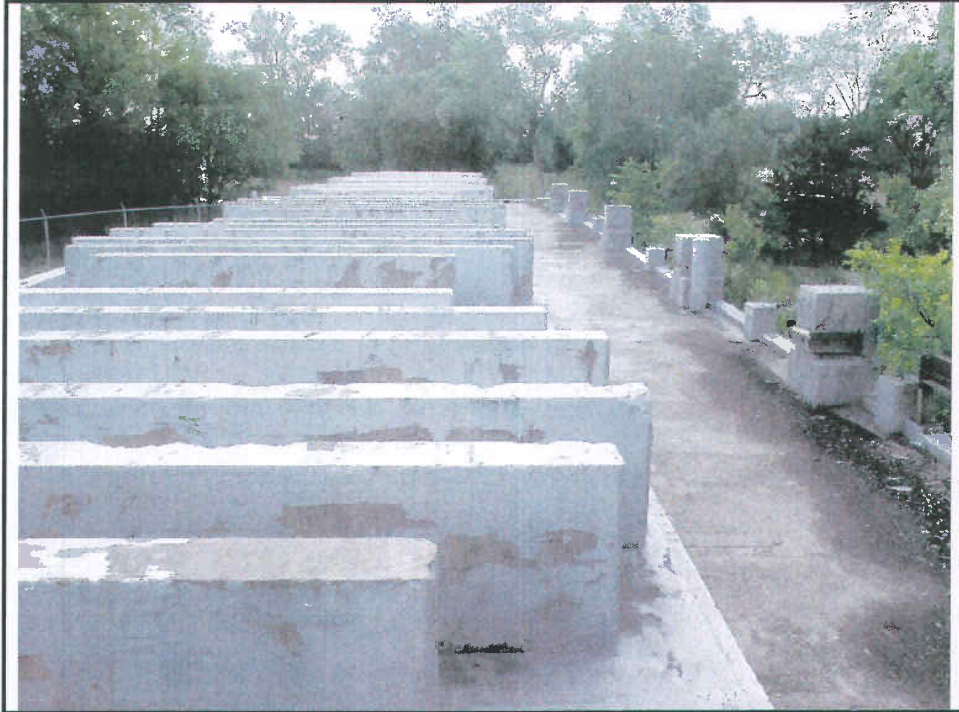
Photo 32: 401-A Power Plant A remnant
