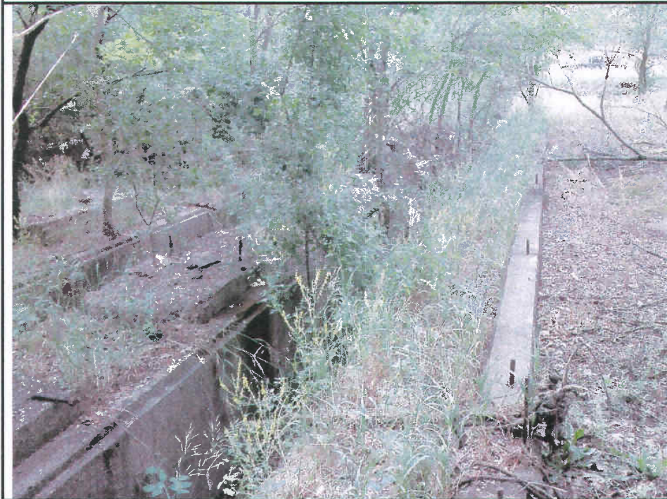
Photo 33: 226-A Hydraulic Refrigeration House remnant (Between A and B Lines)
