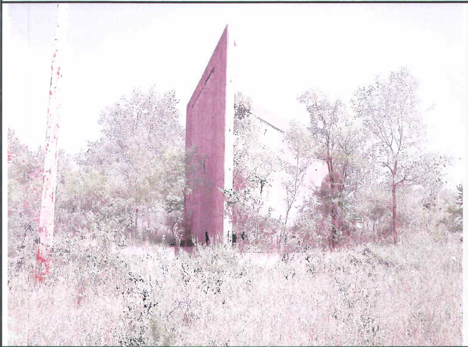
Photo 26: 214 C-11 T-Wall remnant
