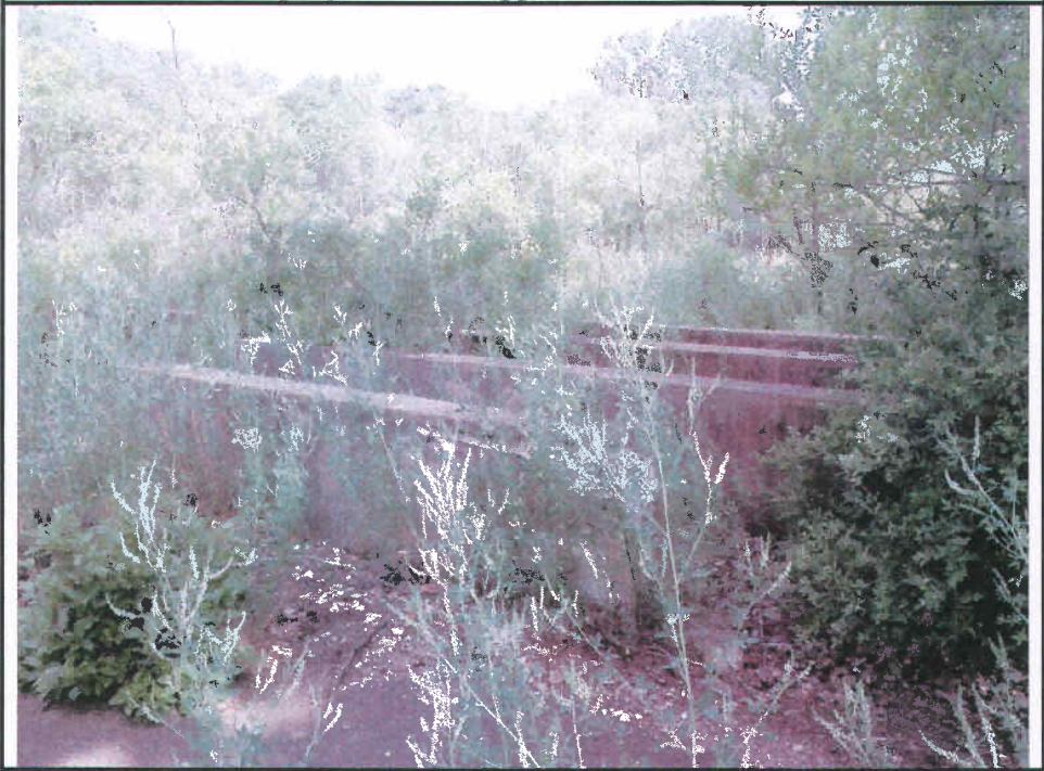
Photo 4: 112-F Poacher Tub House – Support structure
