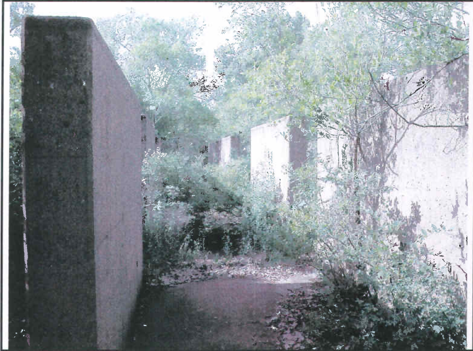
Photo 3: 109-F Pulping House – Support structure
