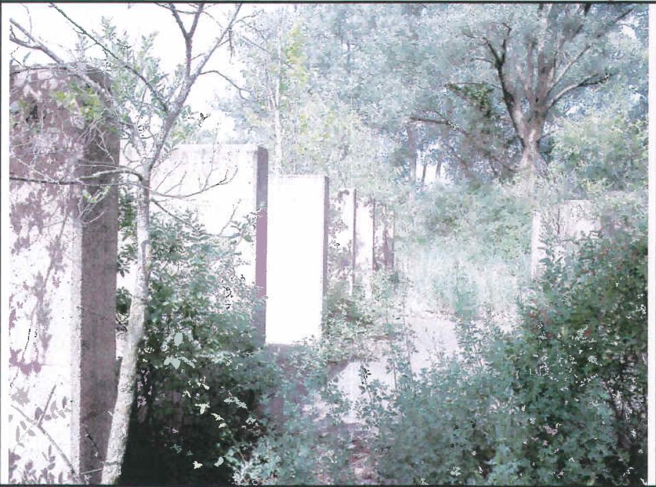
Photo 2: 109-F Pulping House – Support structure
