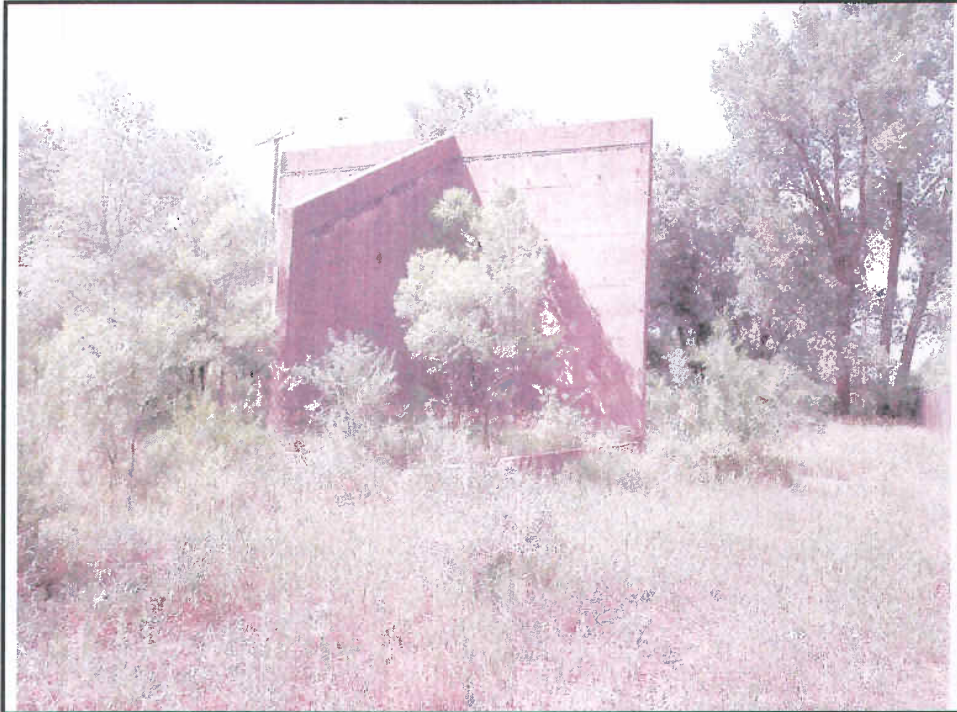
Photo 27: 214 C-11 T-wall remnant
