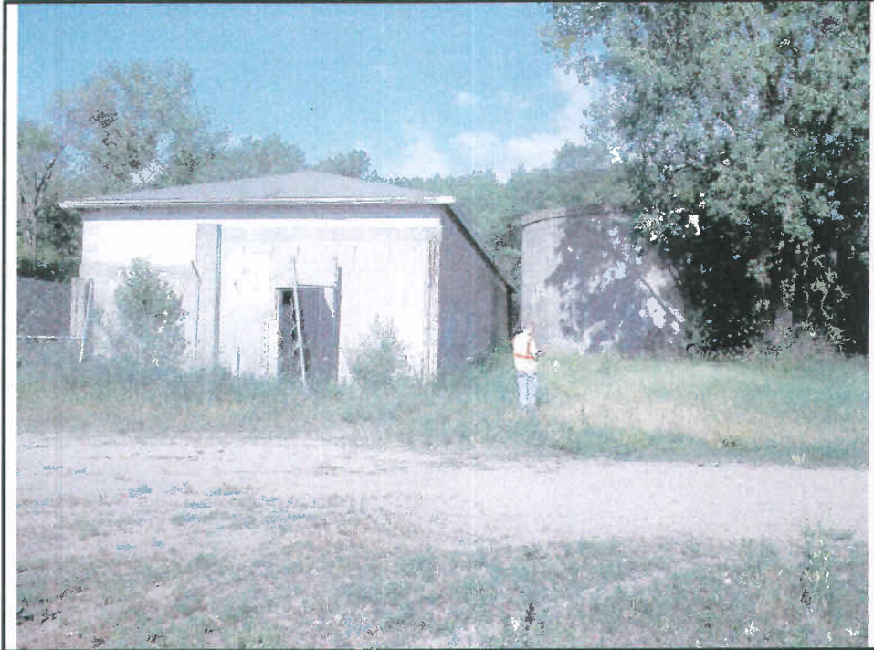
Photo 36: 401-B Power House - Power Plant B
