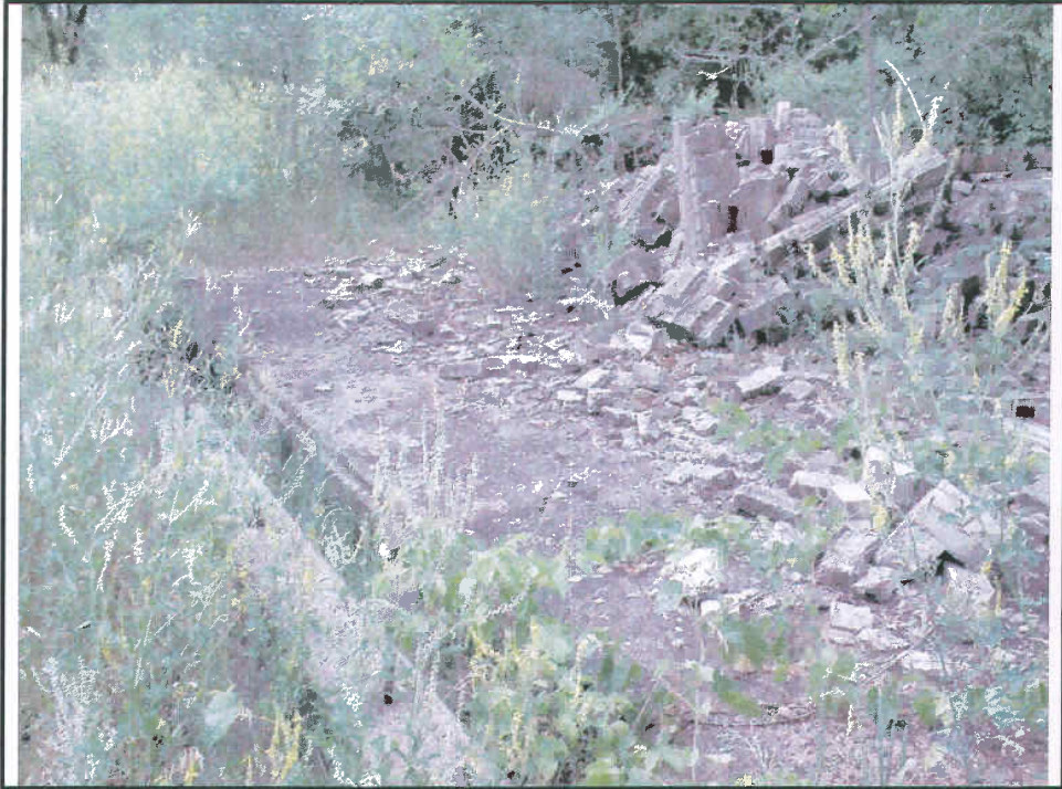
Photo 5: 208-L Mixer House remnant
