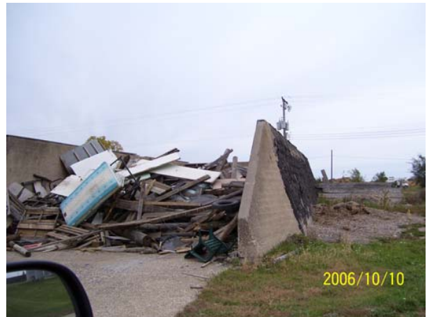
Photo 10. AOC 5. Looking east. DNT storage bunker with trash inside. (1)
