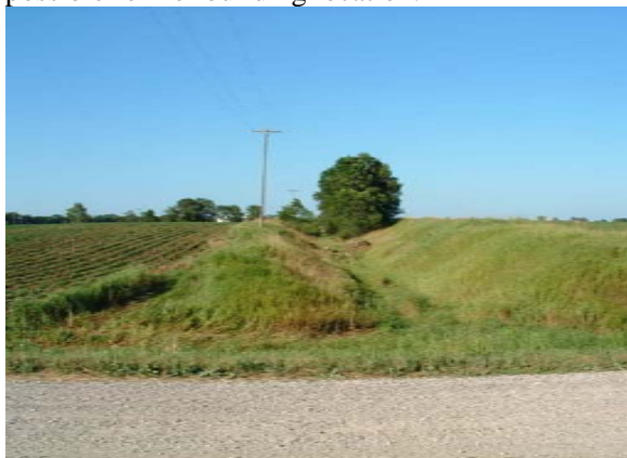
Photo 8. AOC 3, Drainage Area DA1. South and adjacent to AOC 5. (3)
