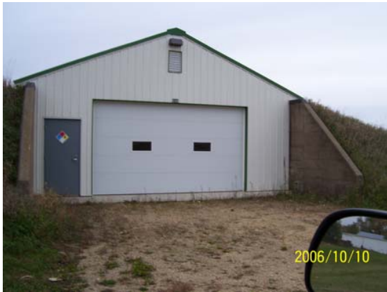
Photo 12. AOC 5. Looking East. DNT storage bunker. (1)
