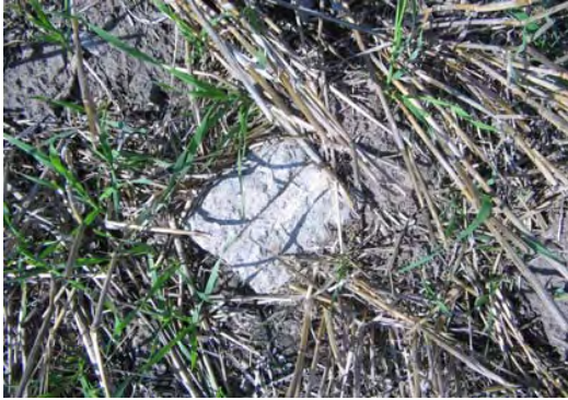
Concrete Debris on West side of 5152 area.
