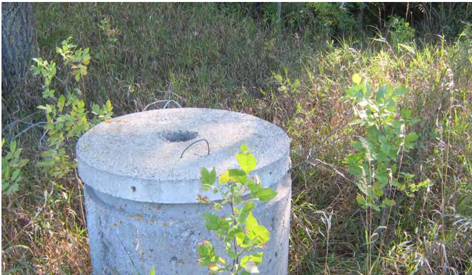
Concrete cistern in former animal waste lagoon west of K street dump area.
