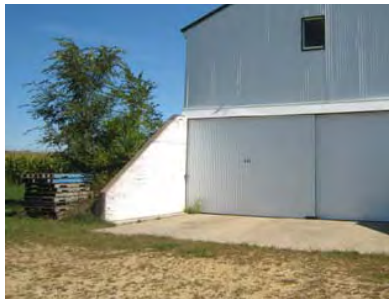
Exterior view of former DNT storage bunker now used for storage.
