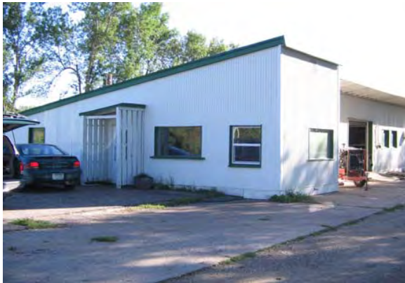
Office building 313 view to east.
