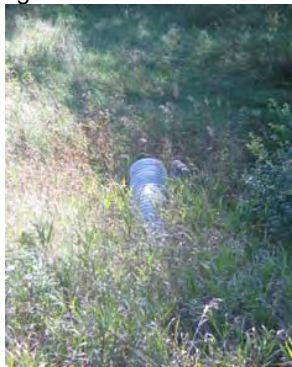
16 inch culvert leading to east basin.
