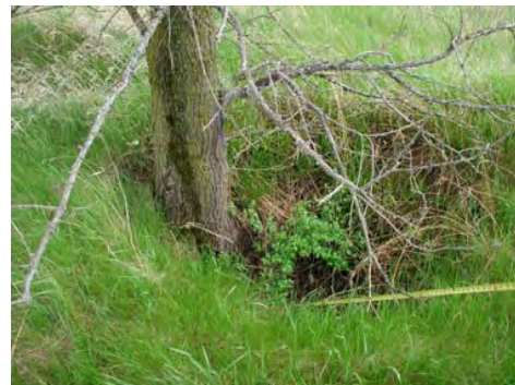
Collapsed Comfort Station 727-K
