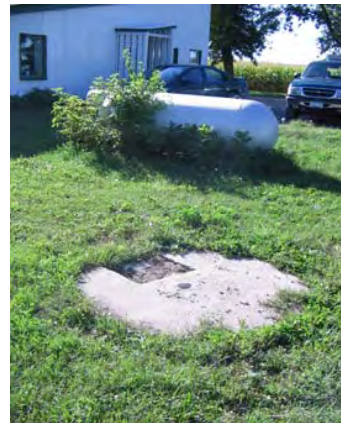
Concrete cistern west of Bldg 313.
