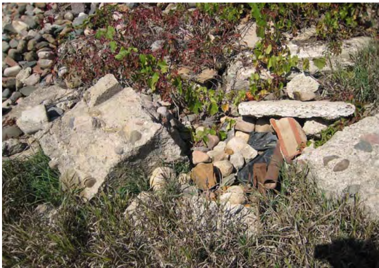
Close up of rubble debris in drainage ditch.
