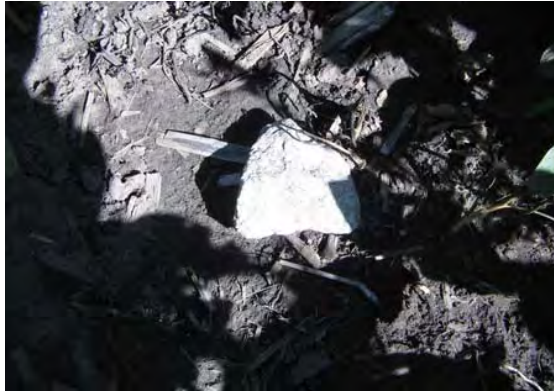
Concrete debris near center of 5152 area.
