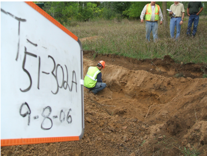
9/8/06: test trench 51 on the southeast corner of the former building pad.
