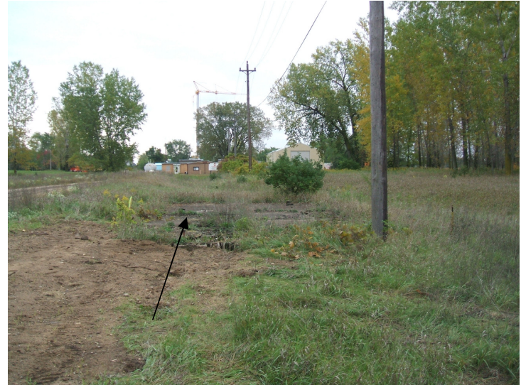
9/23/06: view facing east of concrete building pad.
