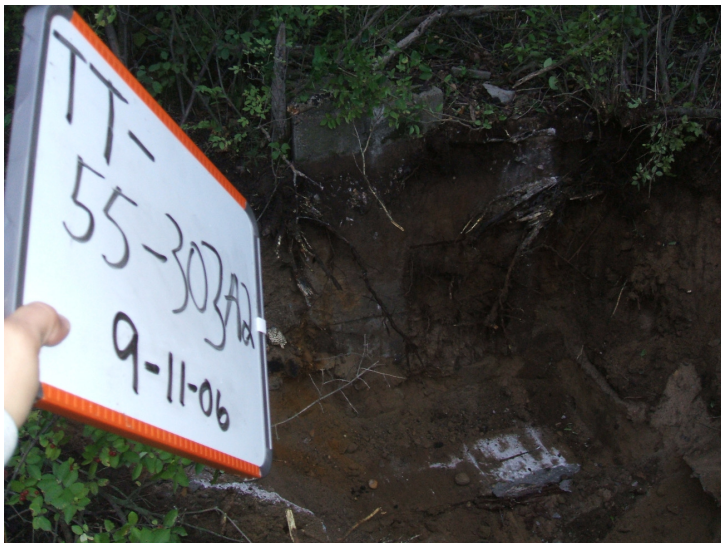
9/11/06: building footing test trench 55 located on southwest building corner.
