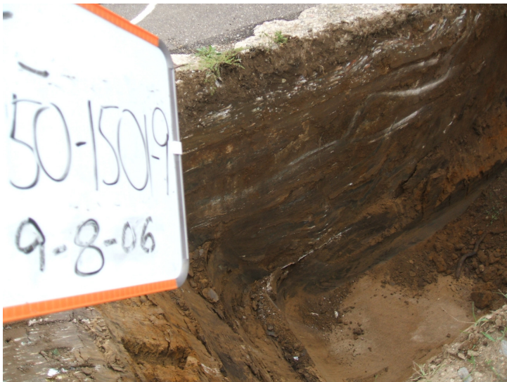
Building 1501-9, test trench 50 located on the west side of the building.
