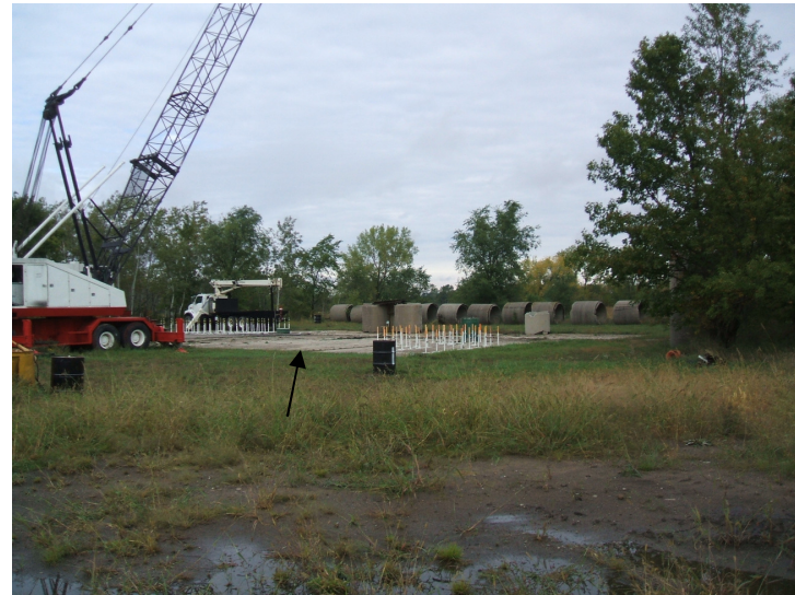
9/23/06: view facing northwest of concrete building pad.
