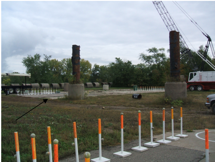
9/23/06: view facing northeast of concrete building pad.
