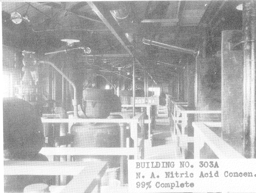
BUILDING NO. 303A N. A. Nitric Acid Concen. 99% Complete
