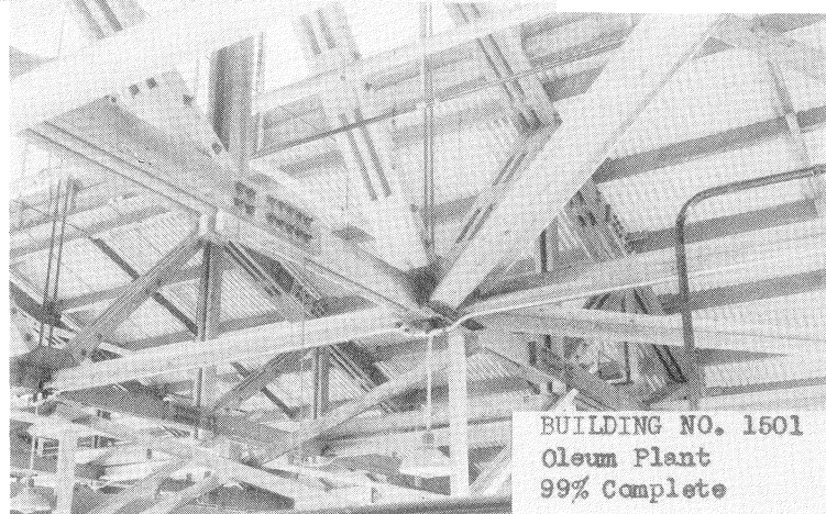
BUILDING NO. 1501 Oleum Plant 99% Complete
