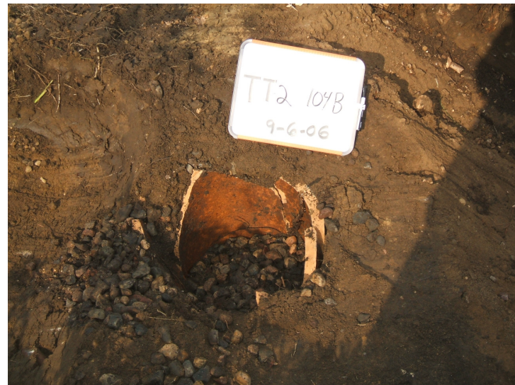
9/6/06: dry well discovered in test trench 2 located a few feet south of the clay pipe that was discovered.
