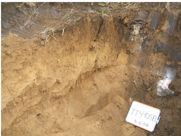
9/6/06: test trench 4 located on the north side of the building.
