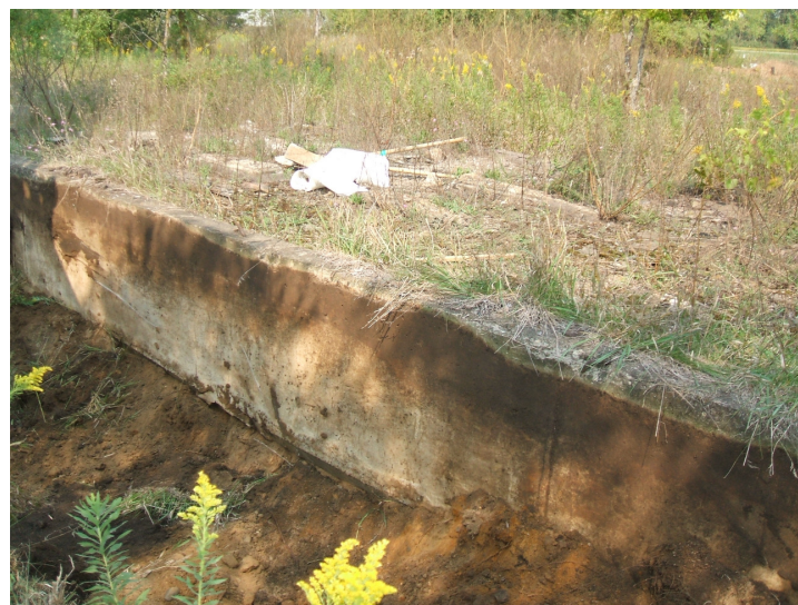
9/6/06: concrete footing along test trench 5 along south side of the building.
