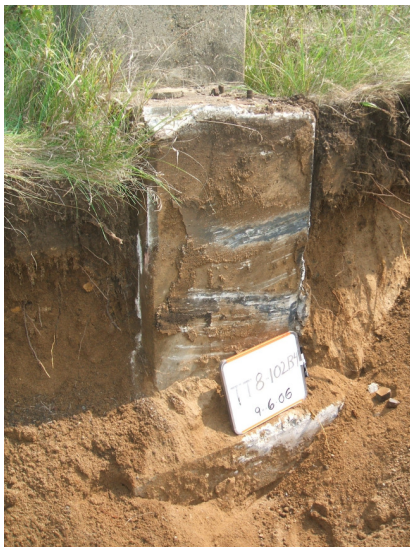
9/6/06: concrete footing in test trench 8.
