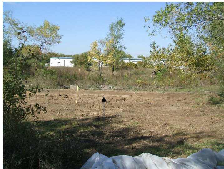
9/20/06: view facing north of concrete building pad.
