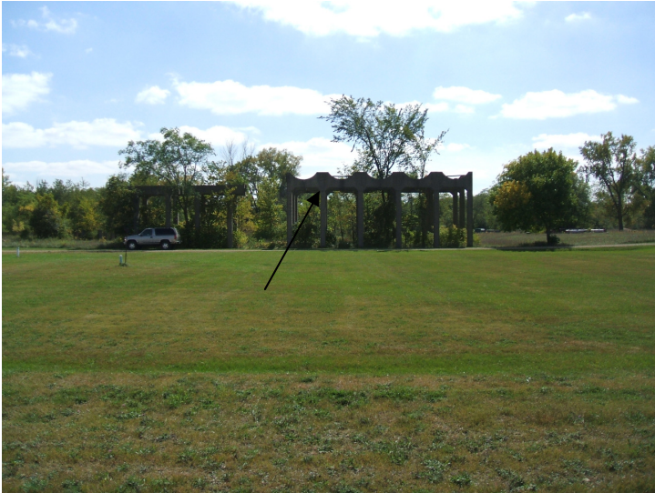
9/20/06: view facing south of concrete remnant of the building.
