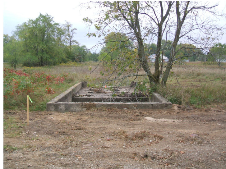
9/21/06: view facing south of concrete building pad.
