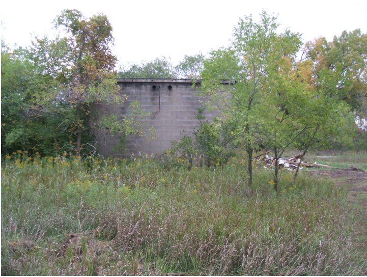
9/21/06: view facing north of building.
