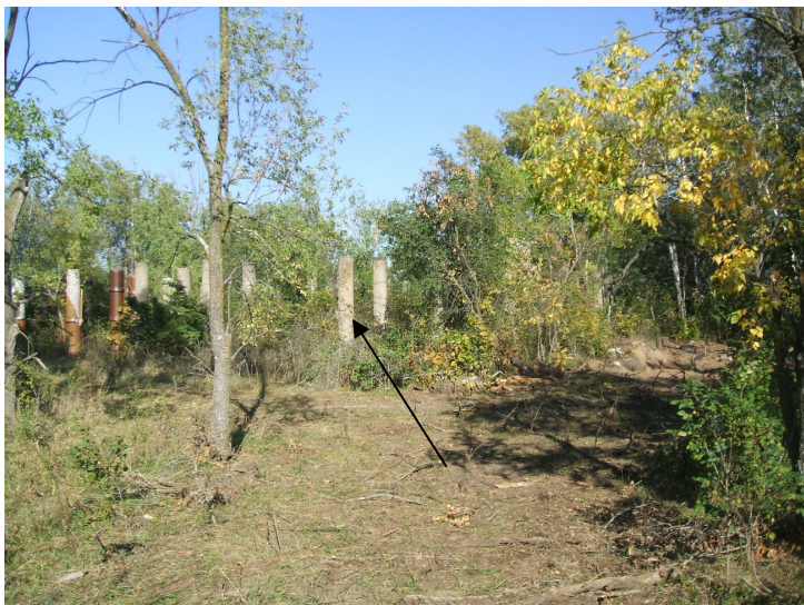
9/20/06: view facing northeast of pillars standing on the concrete building pad.
