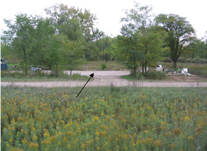
Building 722B, view facing east of the concrete building pad.
