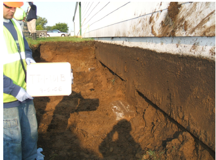
9/6/06: test trench 1 facing west.
