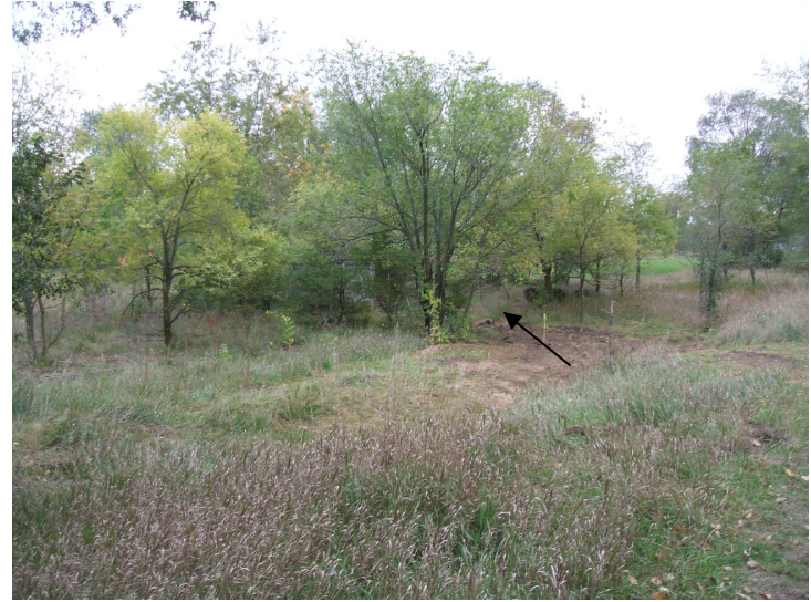
Building 706J, view facing southeast of concrete building pad hidden by trees.
