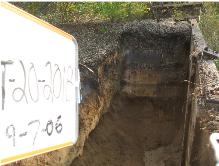
9/7/06: test trench 20 located at the northwest corner of the building.
