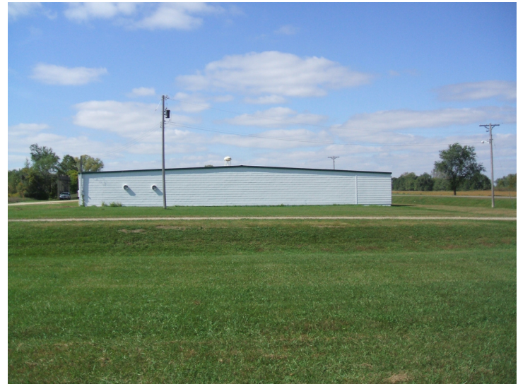
9/20/06: view facing west.
