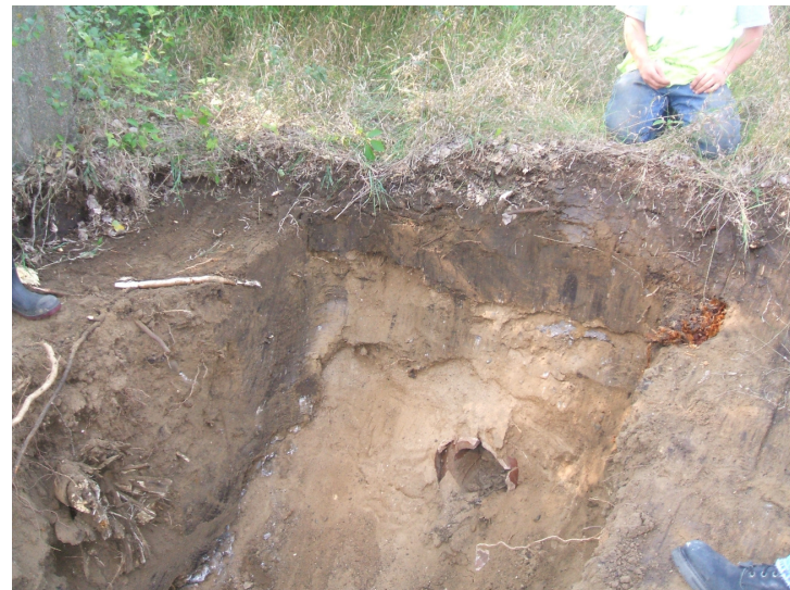
9/6/06: clay pipe discovered in test trench 13 located on the east side of the building.
