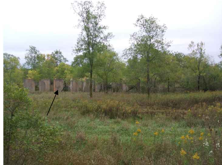
9/21/06: view facing south of concrete supports on the concrete building pad.
