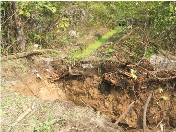
9/6/06: test trench 11 located along the central portion of the west building wall.
