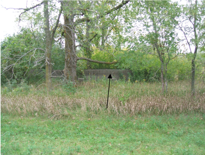
9/21/06: view facing east of concrete building remnant.
