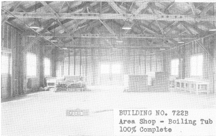
BUILDINGS NO. 722B-BB Area Shop - Boiling Tub 722B-100%, BB-88% Complete
