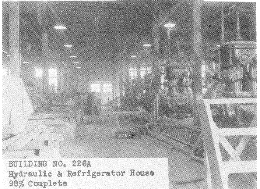
BUILDING NO. 226A Hydraulic & Refrigerator House 98% Complete
