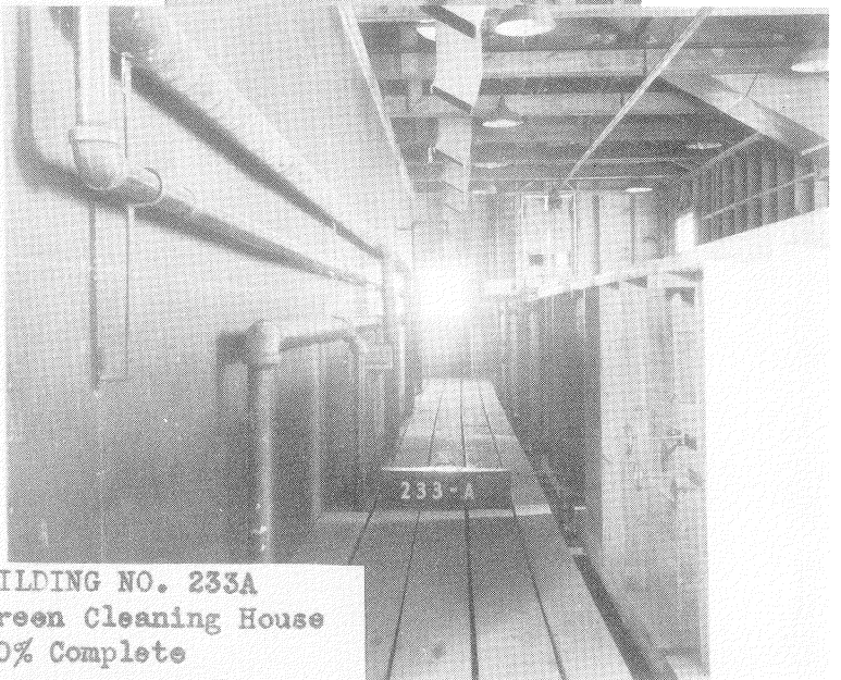
BUILDING NO. 233A Screen Cleaning House 100% Complete
