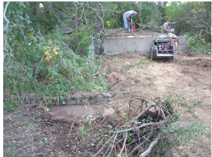
9/15/06 location of concrete sample 56 (working on) and 57 (close flag) on the concrete building pads.
