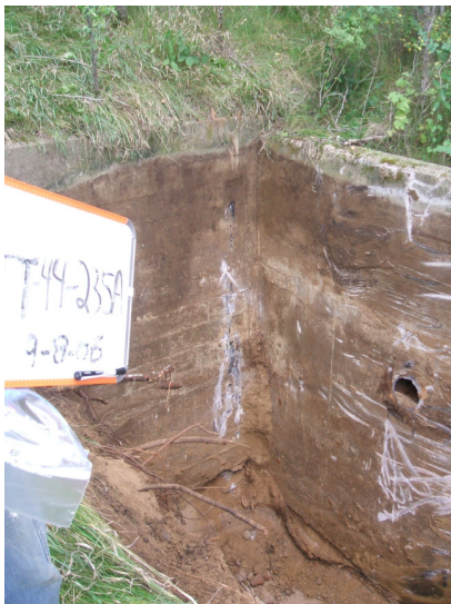
9/8/06: building footing along test trench 44 located along the west building wall.
