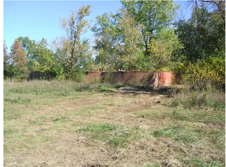
9/25/06: view facing northeast of raised concrete building pad.
