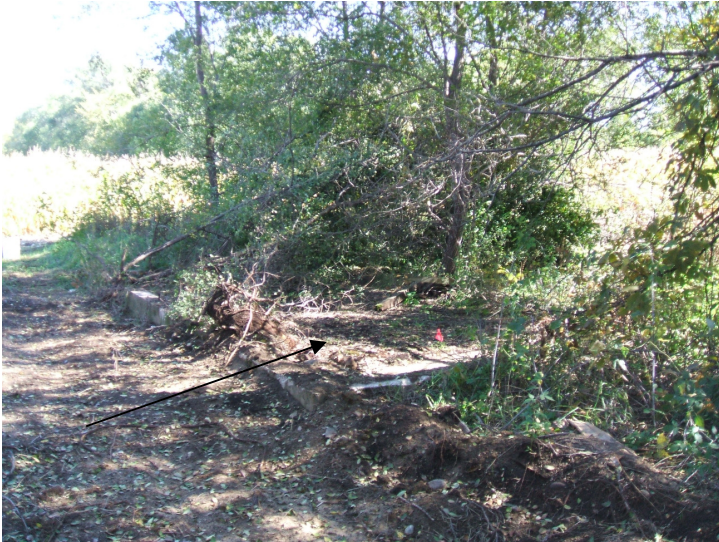
9/25/06: view facing east of concrete building pad.
