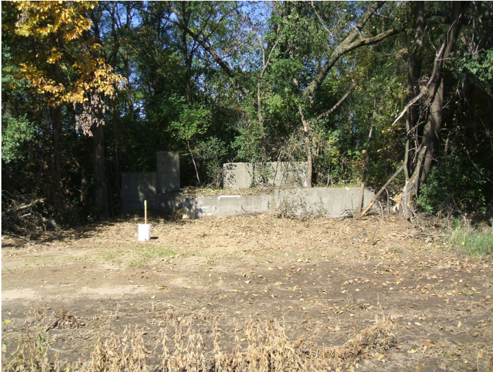
9/25/06: view facing north of raised concrete building pad.
