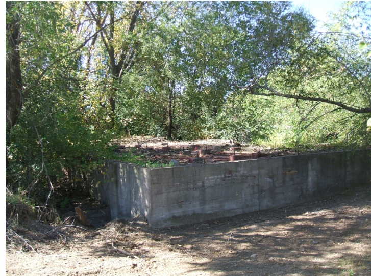
9/25/06: view facing northwest of the raised concrete building pad.
