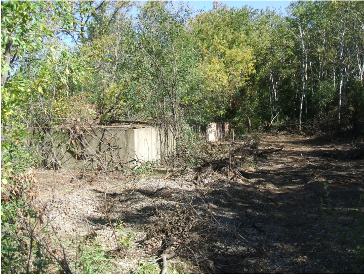
9/25/06: view facing east of raised concrete building pad.
