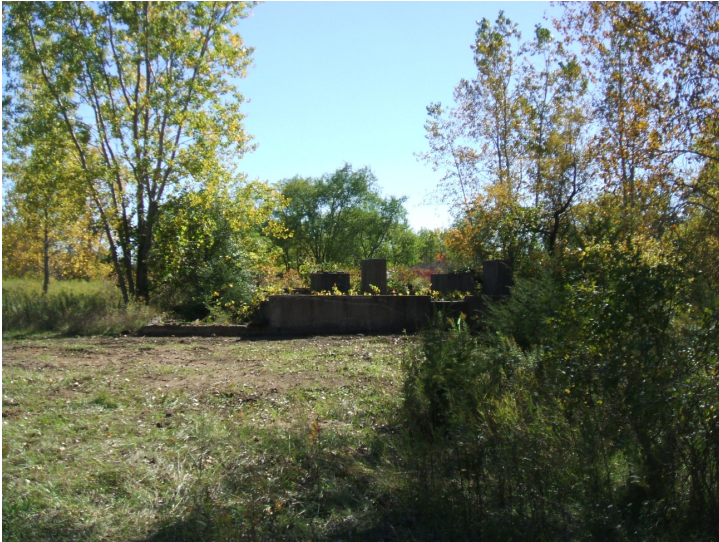
9/25/06: view facing south of concrete building remnants.
