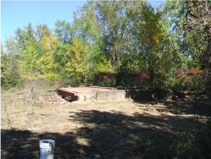
9/25/06: view facing north of concrete building pad.
