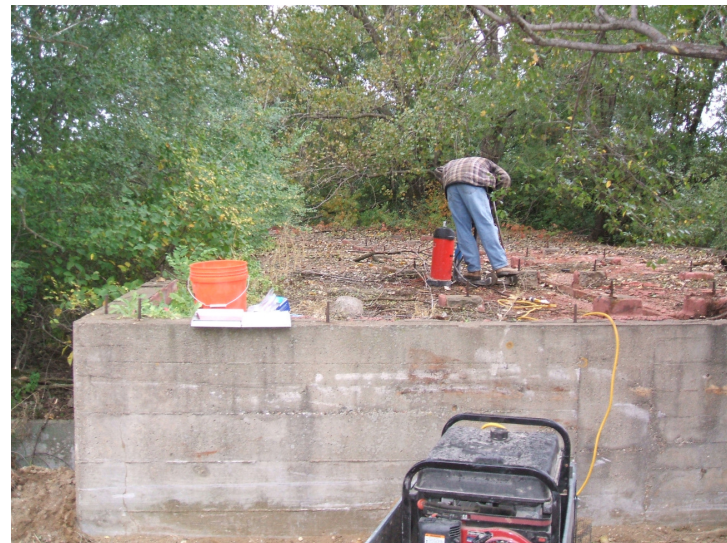
9/18/06: possible ACM red mastic and concrete sample 58 on building pad.
