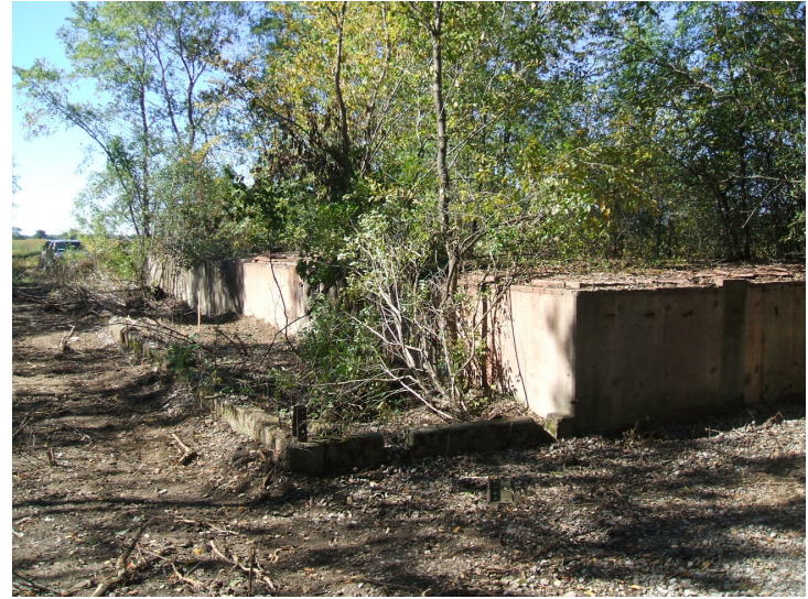
9/25/06: view facing west of raised concrete building pad
