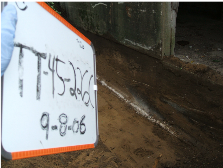
9/8/06: building footing along test trench 45 (building number in photo is wrong) located on the northwest corner of the building.
