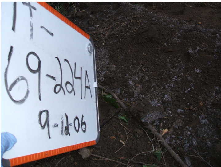
9/12/06: gray material near surface at test trench 69 located on the central portion of the north building wall.
