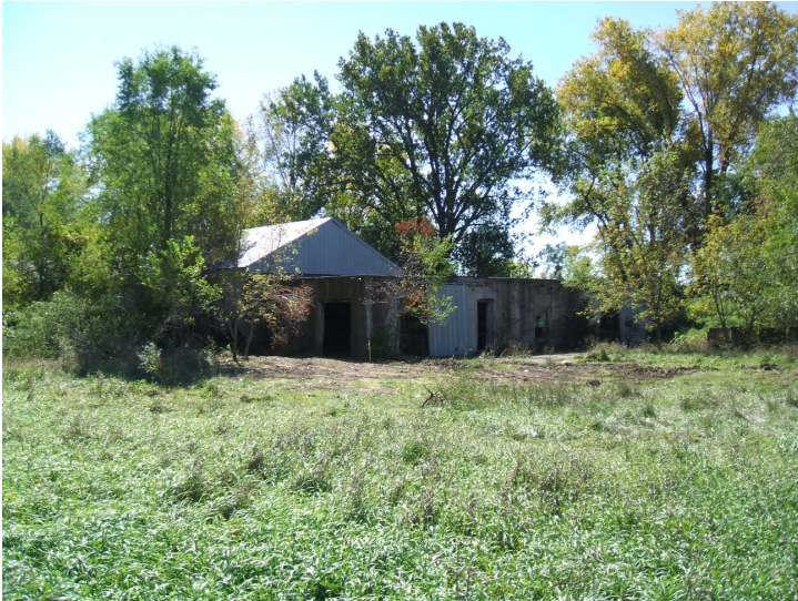
9/25/06: view facing south of building remnant.
