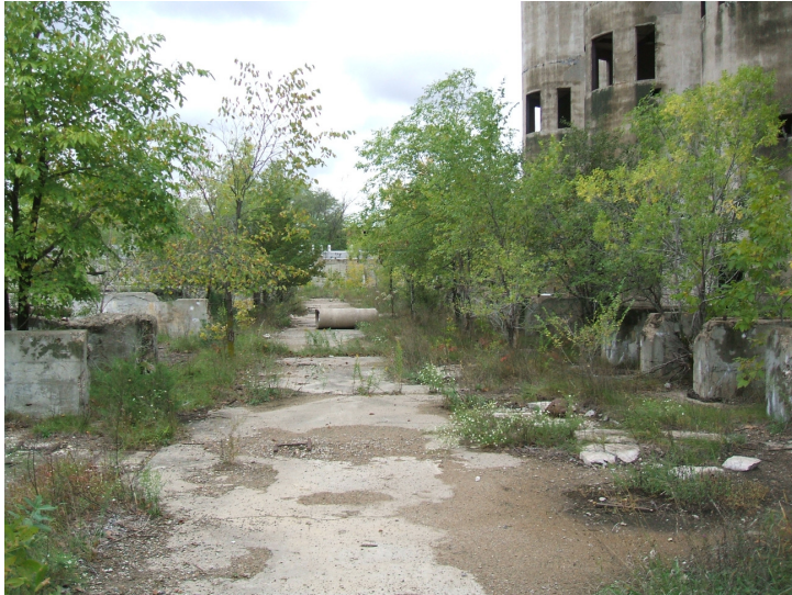
9/23/06: view facing north.
