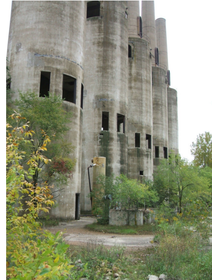
9/23/06: view facing southeast.
