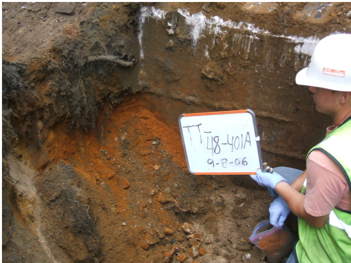
9/8/06: orange stained soil along ash trench in test trench 48 located in the south central portion of the west building wall.
