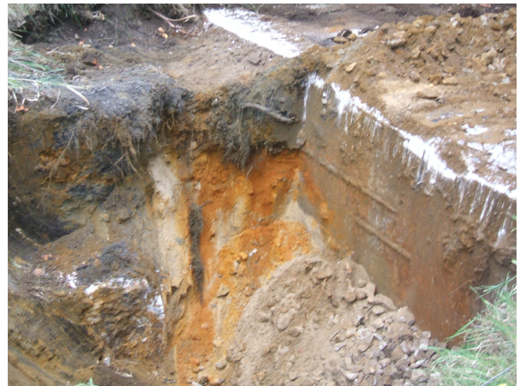
9/8/06: orange stained soil in test trench 48 located in the south central portion of the west building wall.
