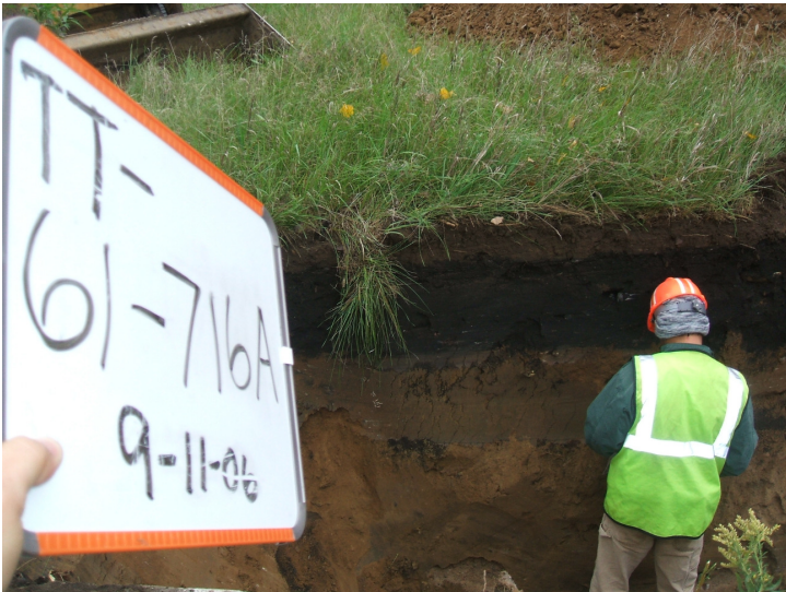
9/11/06: test trench 61 located on the east side of the building.
