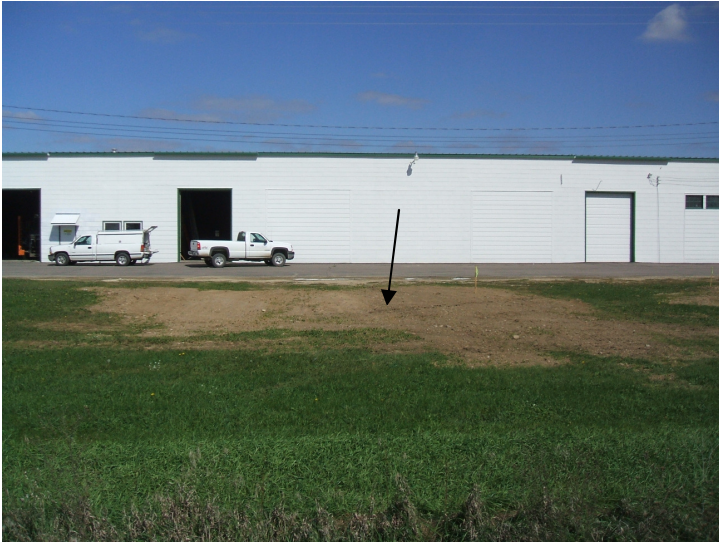
9/20/06: view facing north of former building pad now gone.
