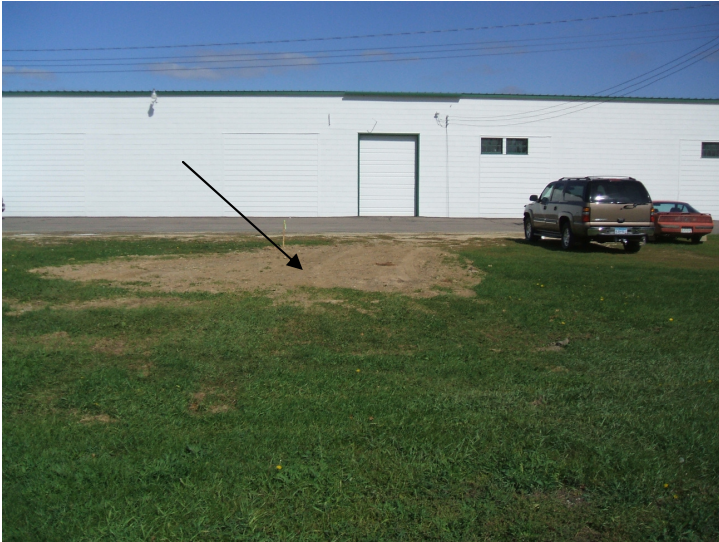
9/20/06: view facing north of former building footing now gone.
