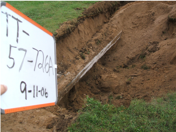
9/11/06: old footing in test trench 57 located inside the east building wall.
