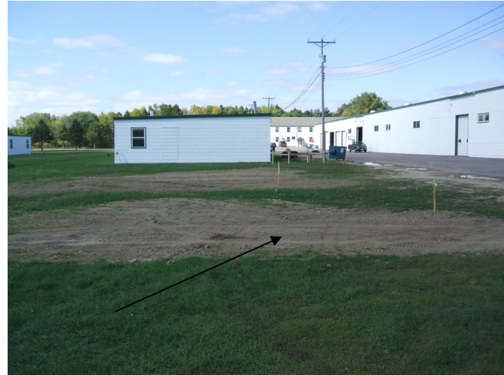
9/20/06: view facing west of former building footing now gone.
