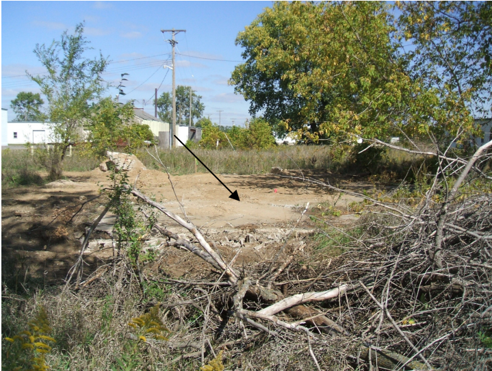
9/20/06: view facing north of the concrete building pad.
