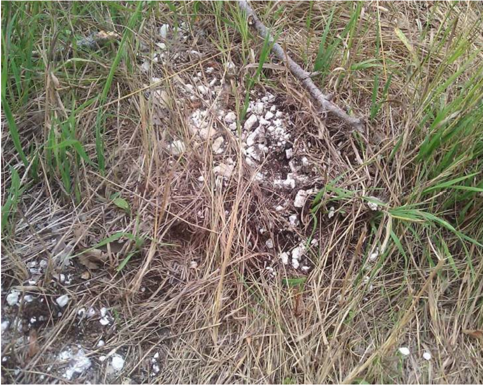
Photo 1: Wallboard at GC-SS4 in GOW Central subarea.
